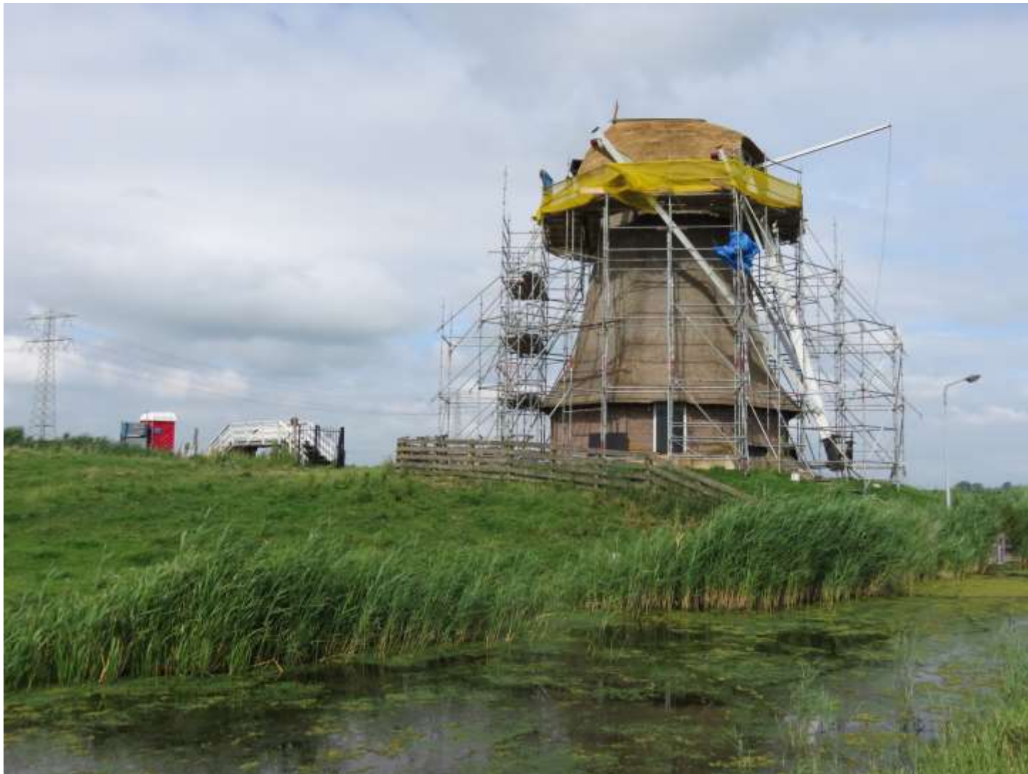
Himpenserpoldermole Wergea, restauratie 2016
